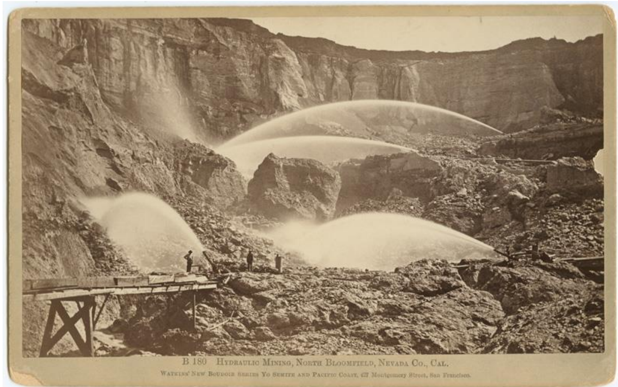
Figure 4: Hydraulic mining North Bloomfield Nevada in the 1880s (California State Library).
